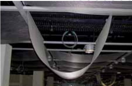
Open position of a woven wire cloth element edged with slotted profiles
