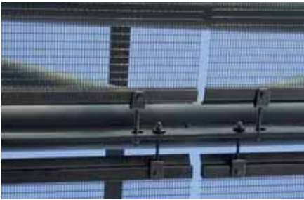
Woven wire cloth elements tensioned using tension profile and clevis screw system
